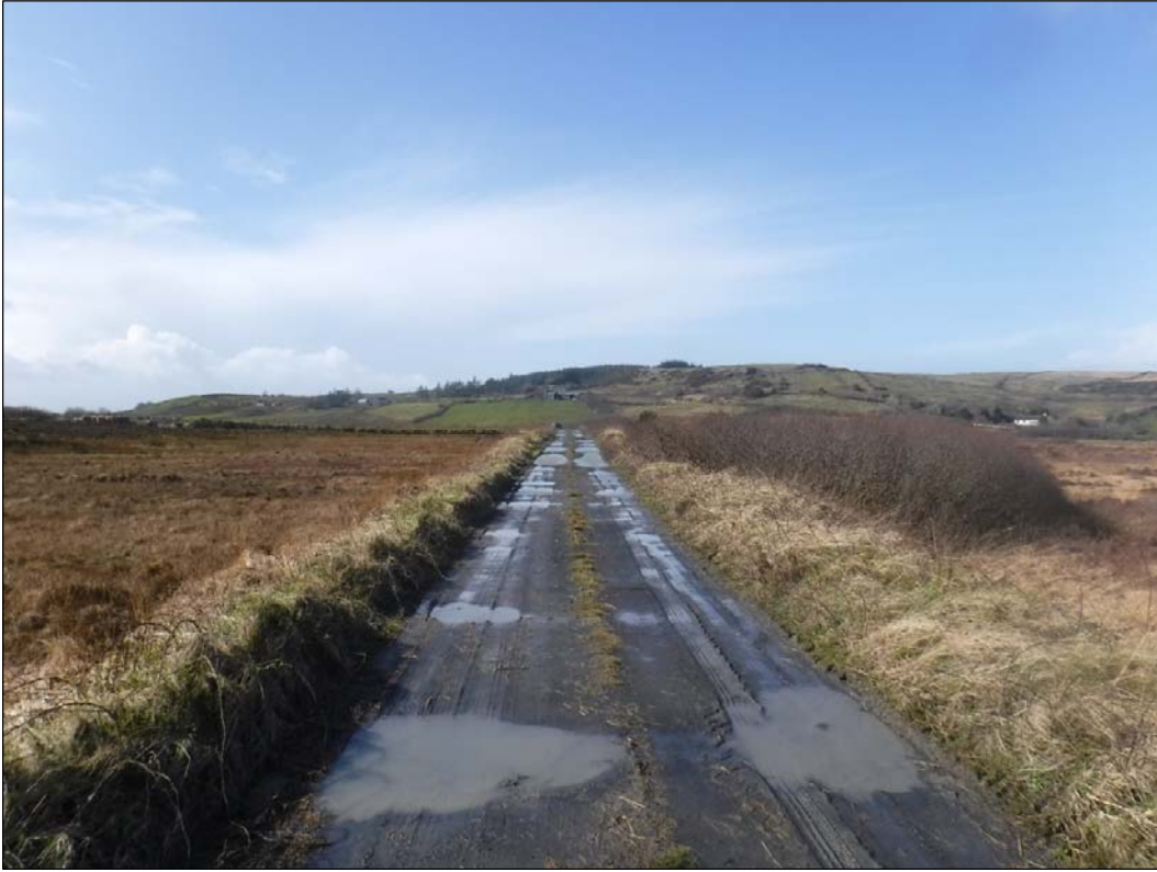
Photo 3: Existing entrance road from north-east of site
